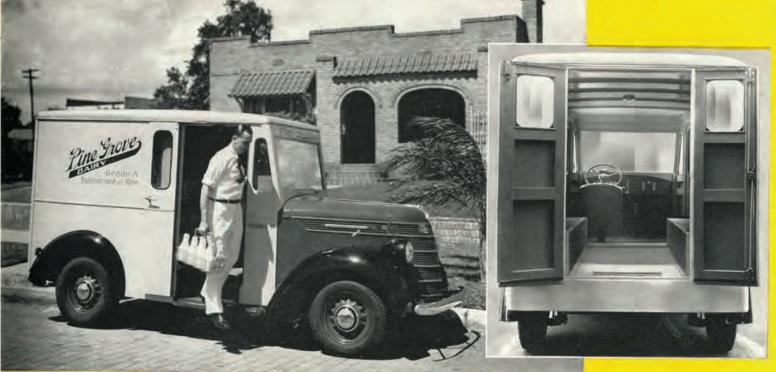
The double rear doors of the type DM and DB bodies, fold back against the body as shown at left. The advantages of this design are ample loading and unloading space, and utility and convenience for work at the loading platform or elsewhere. A solid rear-end construction or three rear doors (shown below) are preferred by some bakers and are available if desired. When used for bakery service the galvanized floor covering is removed and half-round wheelhouses replace the square houses.
